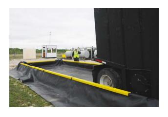
9. Carefully drive/roll container (frac tank, etc) into Containment Wall system.
